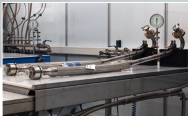
Flushing the piping systems under clean room conditions
